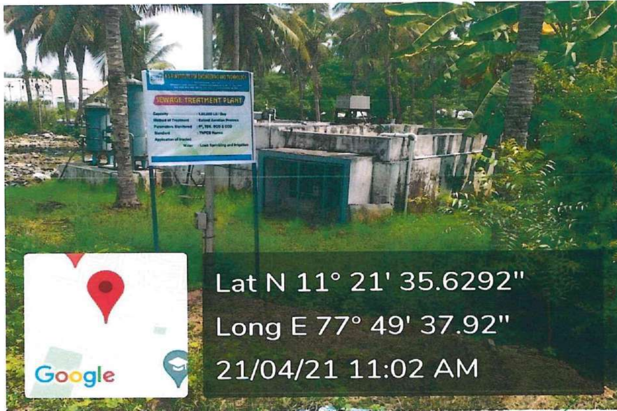
Sewage Water Treatment Plant
