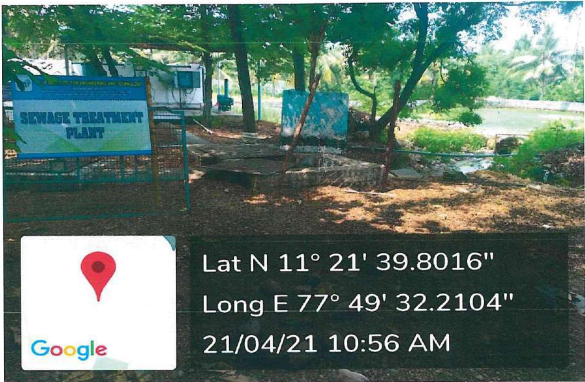
Sewage Treatment Plant
