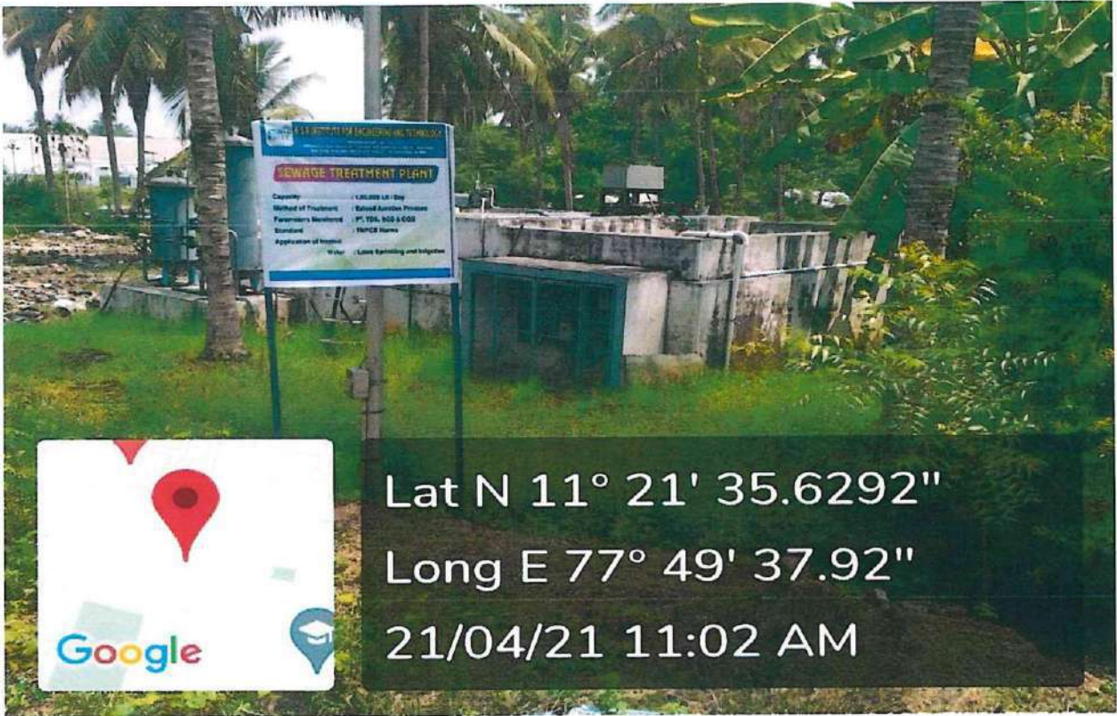
Sewage Treatment Plant
