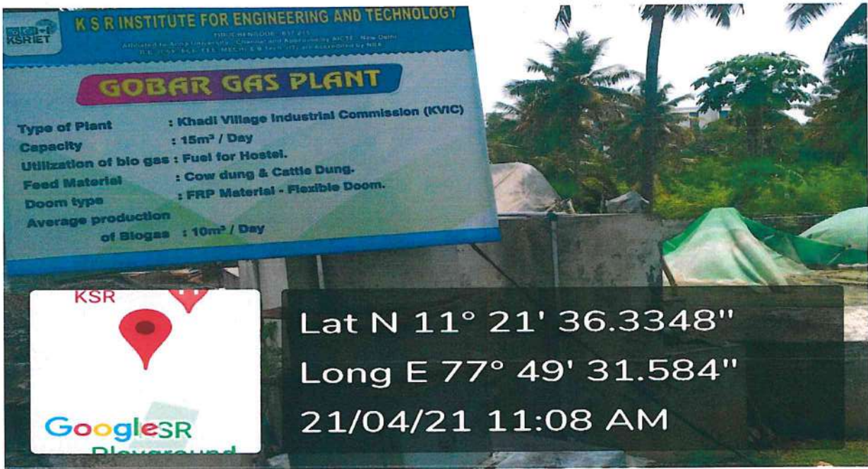
Gobar Gas Plant
