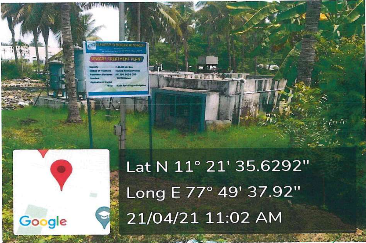
Sewage Water Treatment Plant
