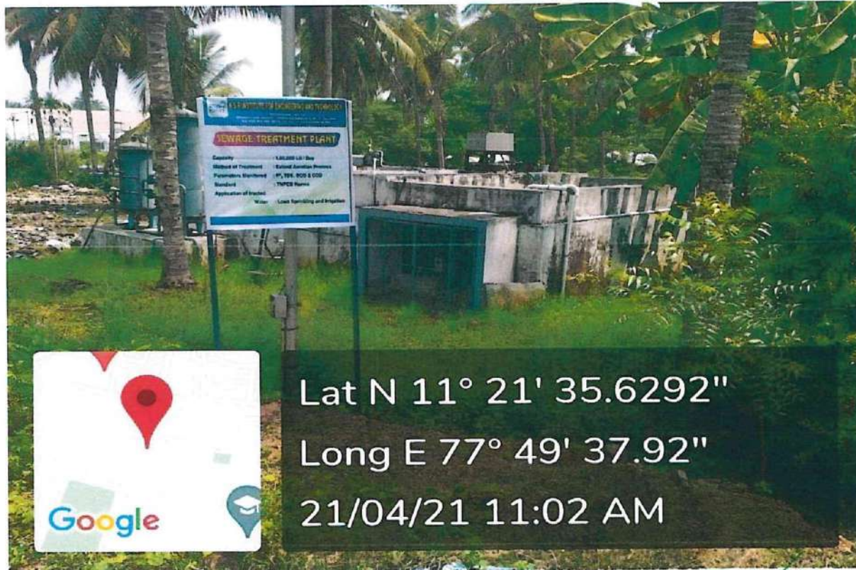
Sewage Water Treatment Plant
